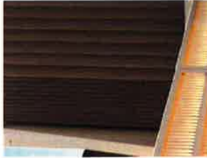
AL 1 VERTICAL BRONZE ANODIZED ALUMINUM LOUVERS
